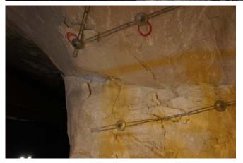
Steel straps are not really suitable to provide a confinement.
