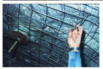
Steel mesh may be an alternative to provide a confinement.
