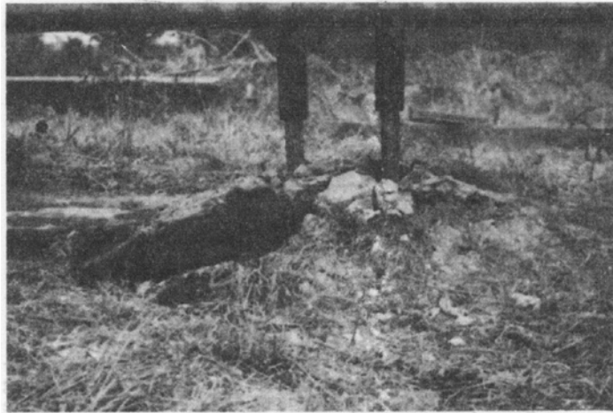
Fig. 1b. After Failure View of a Group of Two Anchors
