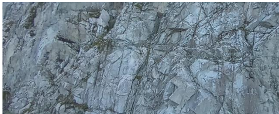
Figure 3: Fjord of Puyuhuapi – Highly fractured rock mass
