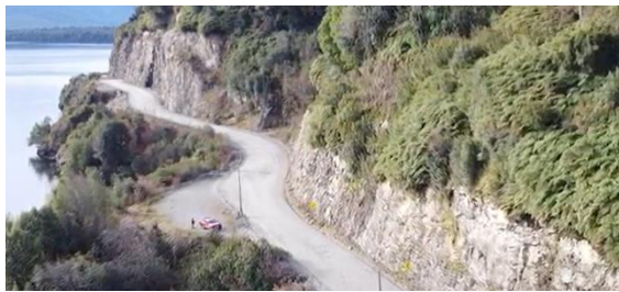
Figure 2: Fjord of Puyuhuapi – Location of the most difficult slope
